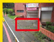
女生宿舍L棟 Girls Dormitory Building L
